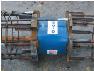
Figure 4 – O-cell Installed in Rebar Cage
