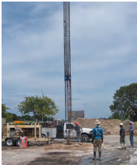
Figure 5 – Installing Rebar Cage in Test Pile
