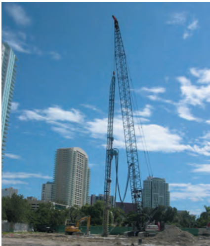
Figure 3 – ACIP Piling Installation
